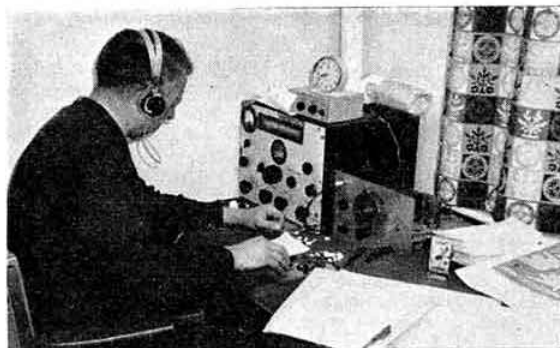
G3FM operating on behalf of the Reigate Amateur Transmitting Society during the Affiliated Societies' Contest in February, 1962. G3NKS also operated while G3NKT and G3PIJ acted as logkeepers. The equipment included a CR100 receiver, v.f.o./buffer/807 p.a. transmitter and a half-wave aerial at 40 ft.
